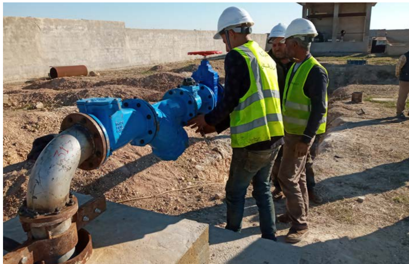
Water pump repairs at the Allouk water station in Syria.
